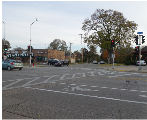
Ludington Avenue intersection. This view from the northwest corner shows the diagonal offset of the Ludington Avenue leg.
