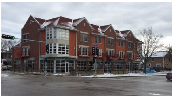
Swan Boulevard mixed use building uses roofline and gables, careful window placement, and variation in height to increase compatibility of a three-story building in its residential context.
