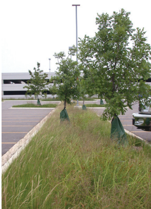
Fig. SSD-9: Bioswales within parking lots can collect stormwater and break up large areas of impervious pavement, Tellabs Corporate Headquarters, Naperville, Illinois.
