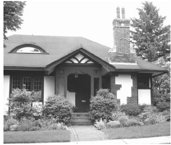
Figure 38: 6437 Upper Parkway North.
