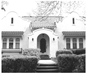
Figure 27: Arched entry at 6913 Grand Parkway.
