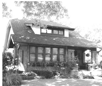
Figure 40: 6235 Upper Parkway North.
