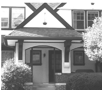
Figure 60: 7429 Hillcrest Drive entry, note the large brackets.
