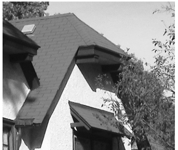
Figure 22: Clipped gable roof at 836 N. 67th Street.
