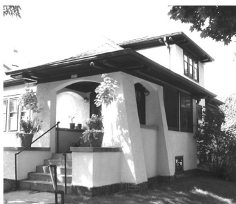
Figure 74: 2379 N. 64th Street.
