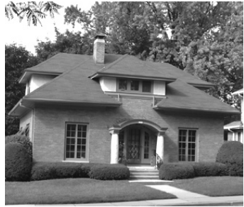
Figure 39: 6301 Upper Parkway North.
