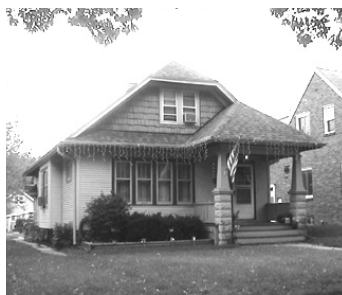
Figure 73: 2425 N. 64th Street.
