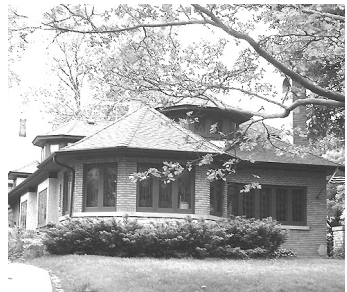
Figure 46: 2183 N. 74th Street.
