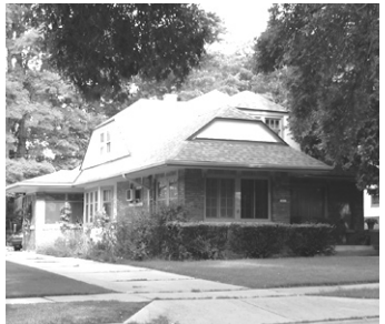
Figure 34: 1821 N. 60th Street.
