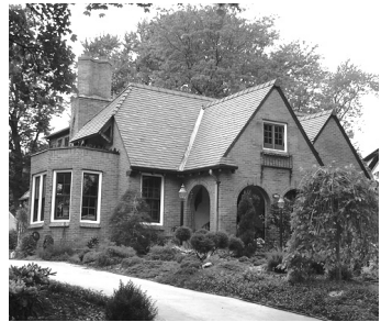
Figure 45: 2169 N. 74th Street.
