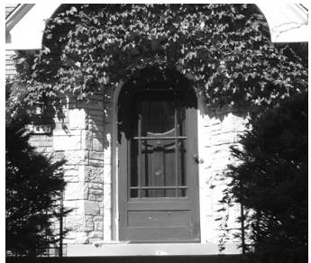
Figure 65: Entry door at 2457 Lefebber Avenue.
