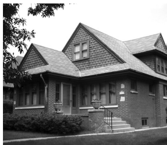
Figure 80: 2450 N. 64th Street.
