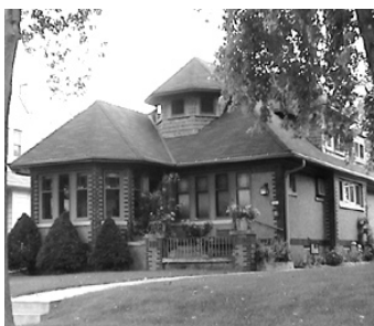
Figure 79: 2462 N. 64th Street.
