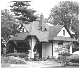
Figure 61: Garage at 7429 Hillcrest Drive.
