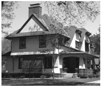
Figure 21: 836 N. 67th Street.
