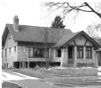
Figure 36: 6514 W. Lloyd Street.
